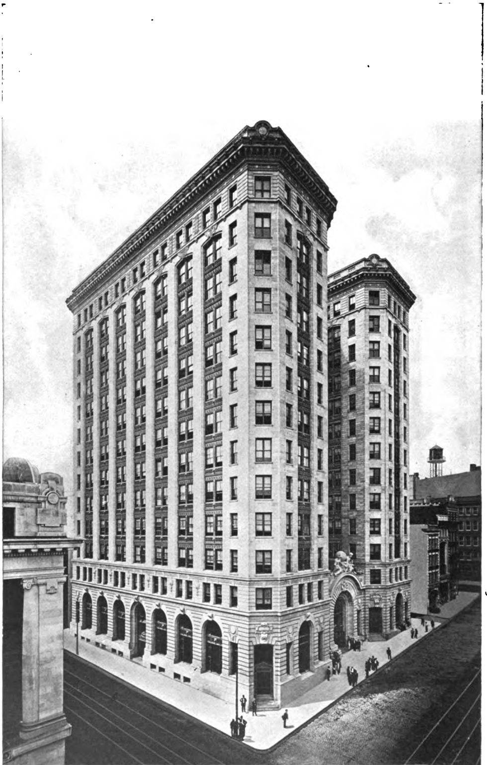
General Office Building Baltimore & Ohio Railroad Company.
